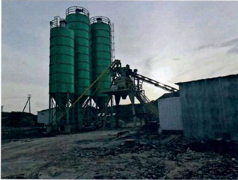
P9: View of Batching Plant
