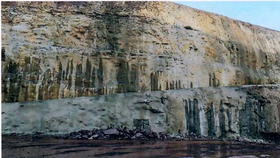
P3: View of Side ramp and Wall of Forebay
