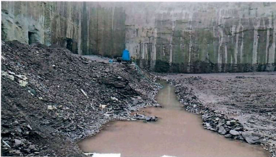
P5: Closure View of Pump house Pit
