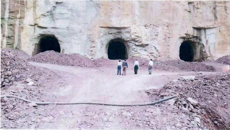
P6: Closer view of Pipe line /Delivery Main Tunnel
