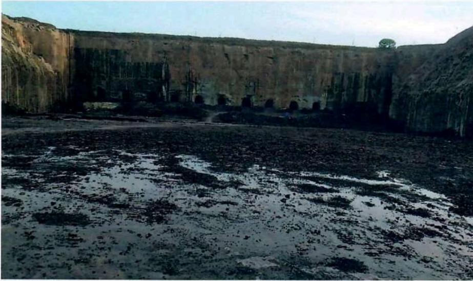
P4: View of Pump house from Forebay
