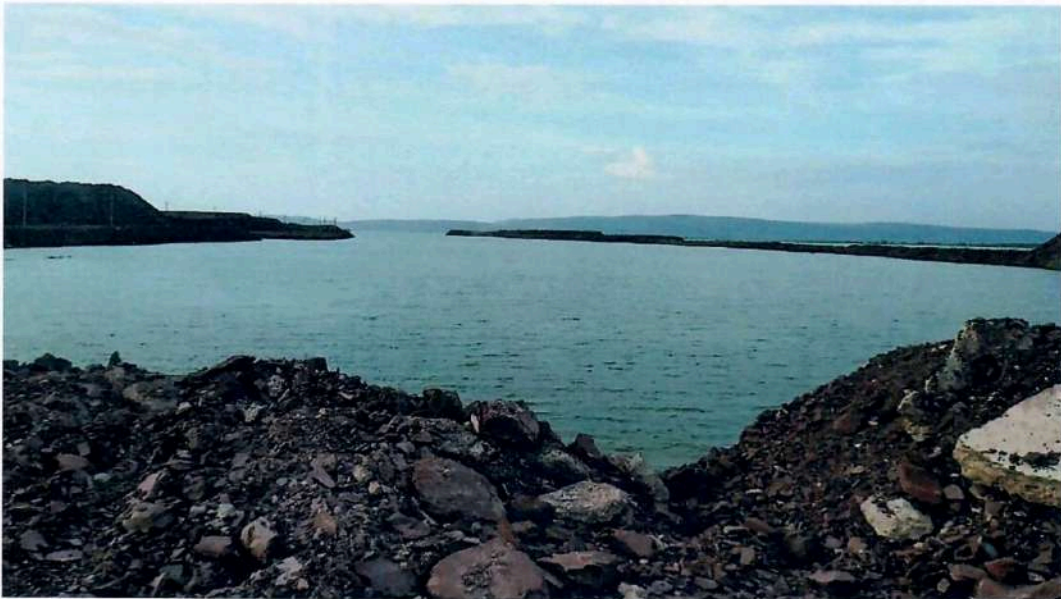
P1: View of Upstream View of the Approach Channel
