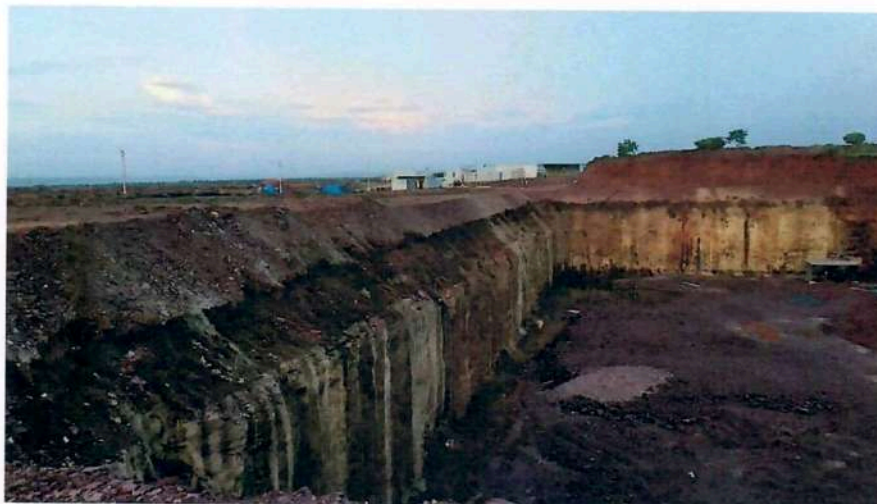
P11: Sheds near upstream side of Delivery Chamber
